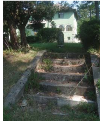
Figure 2. Stairs – constructed elements that are part of the garden initial planning (own source).
