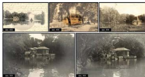
Figure 11. The first wharf (www.googleimages.com; www.googleimages.com; www.only-romania.com; www.only-romania.com; www.only-romania.com)
