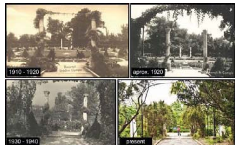
Figure 31. The Rotunda - before and after ( www.googleimages.com ; www.googleimages.com ; www.googleimages.com ; www.googleearth.com )
