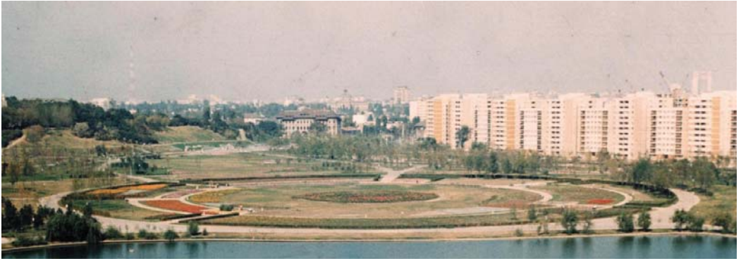
Figure 9. Tineretului Parc – the circular rosarium in the time of its construction (arch. V. Donose archive)
