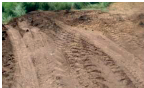
Figure 3. Covering the soil surface with the soil resulting from excavation
