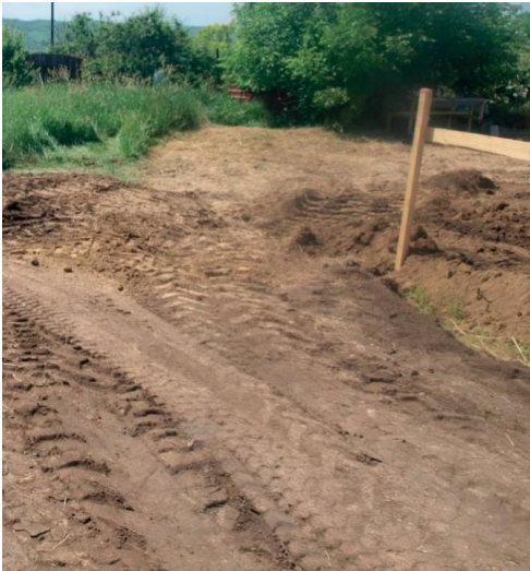
Figure 2. Covering the surface of the land with subsoils material followed by strong compaction
