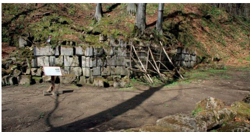
Figure 15. a. The pentagonal tower: photograph from the University Babeş-Bolyai archives (1960s) b. Current image: pressure created by trees on the wall and the destabilization of the terrain edge under the trees' weight are both visible. Source: personal archives (2018)
