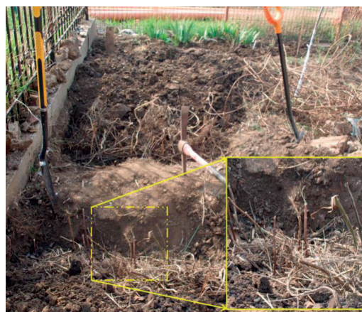
Figure 5. Reclamation works of the strong compacted Urbic Technosols by soil loosening and incorporation into the soil of the plant stems for providing vertical drainage
