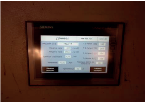
Figure 4. System for monitoring and setting of modes management of the pyrolysis installation
