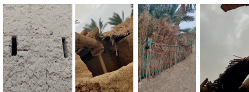
Figure 3. Different applications of palm trees include their use: lintels, beams, fences and false ceilings (Source: Authors, 2018)
