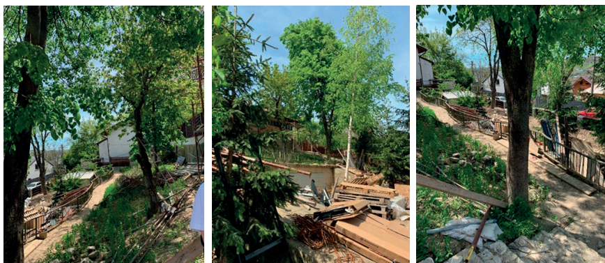
Figure 3. The existing situation of the slope behind "Bojdeuca Ion Creangă" Museum
