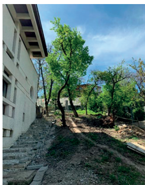
Figure 4. The existing situation of the slope behind "Bojdeuca Ion Creangă" Museum
