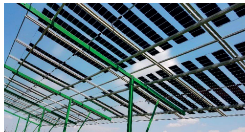
Figure 2. Hortivoltaic two types of semi-transparent photovoltaic panels
