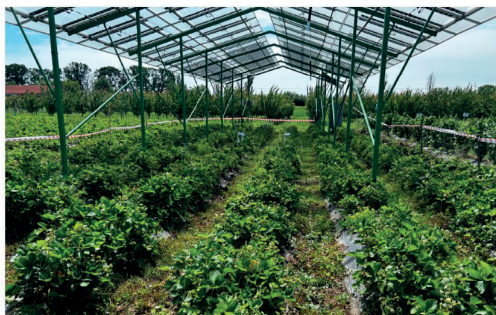
Figure 1. Hortivoltaic system above the strawberry rows
